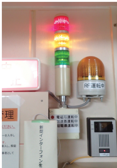
Figure 6-3: Three-color pilot lamp; Red: high voltage, high magnetic field; Green: high pressure gas (Liquid He) ; Yellow: radiation (accelerator operation).
